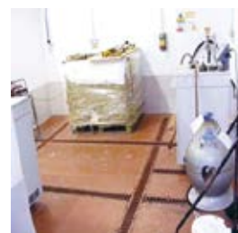
Test Cell with blast walls
